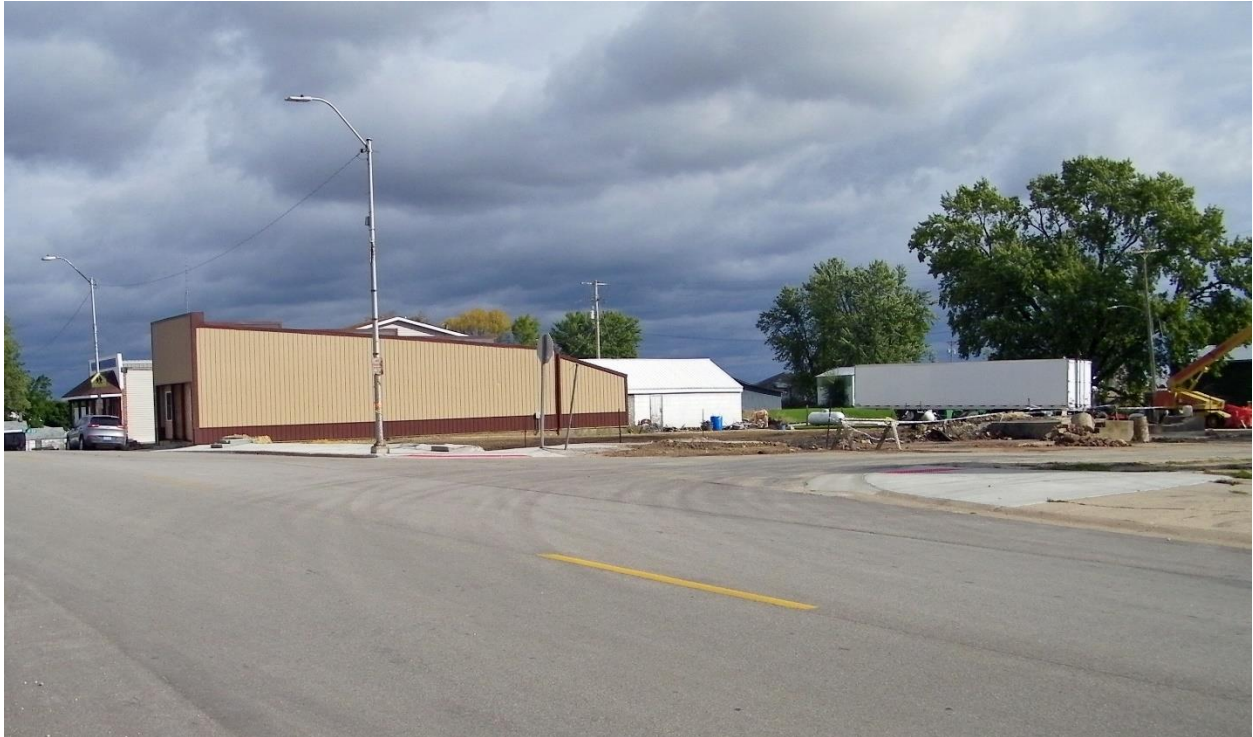
East side of Main Street after the 2019 fire
